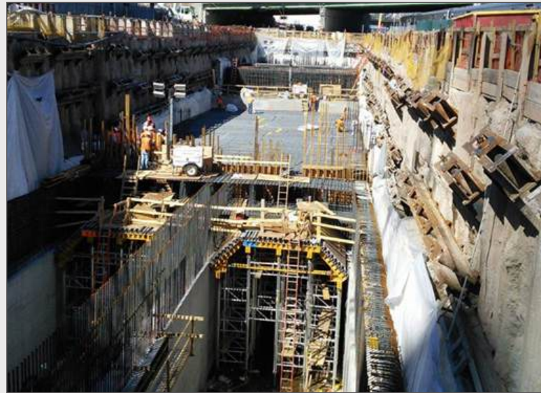
Figure 4-28 Hudson Yards Concrete Casing Project
