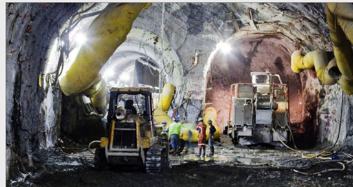
Figure 4-22 TBM Excavation Widening for Cavern Development
