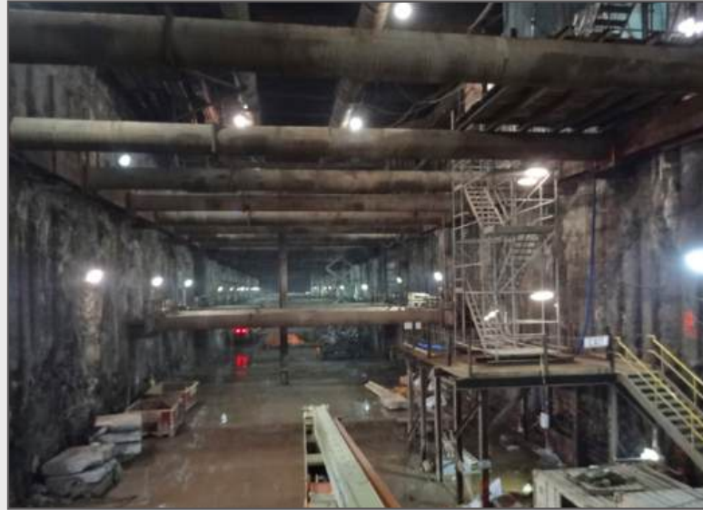
Figure 4-26 Cut-and-Cover Struttred Excavation, Second Avenue Subway Project
