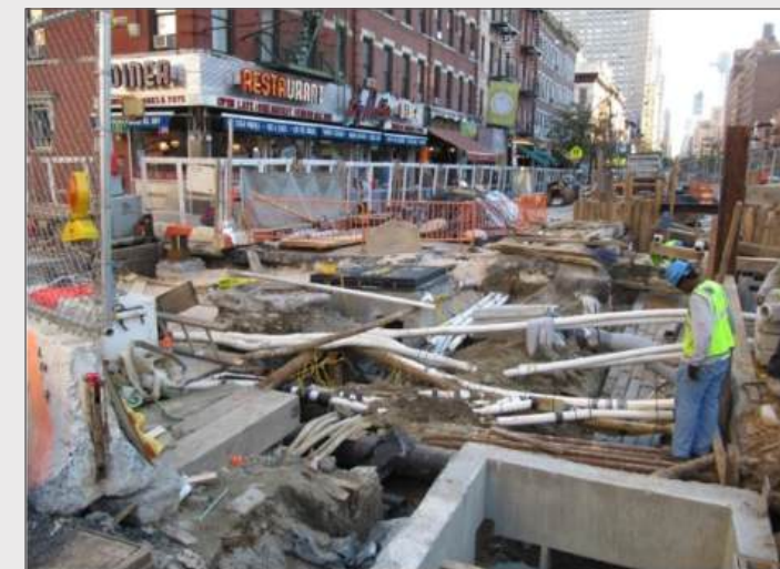
Figure 4-25 Construction in the Street, Second Avenue Subway Project
