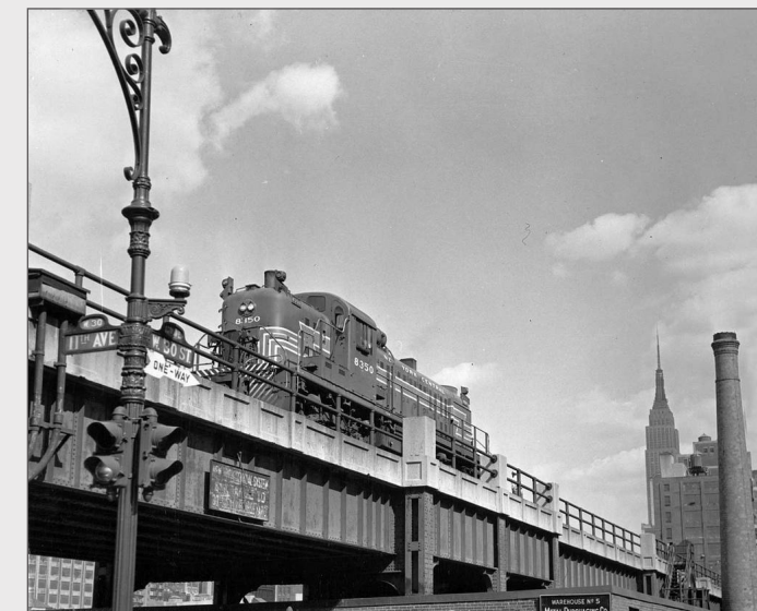
Figure 4-3 High Line in Operation (Eleventh Avenue and West 30 th Street)
