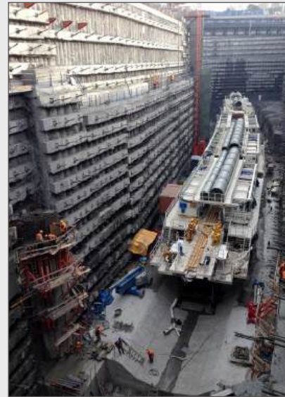
Figure 4-29 Cut-and-Cover Portion of Eurasia Tunnel, Istanbul, Turkey
