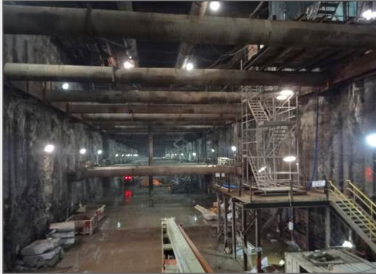
Figure 4-26 Cut-and-Cover Strutted Excavation, Second Avenue Subway Project
