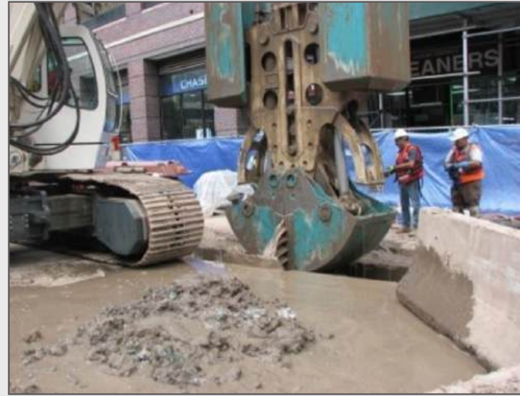
Figure 4-27 Slurry Wall Construction Second Avenue Project
