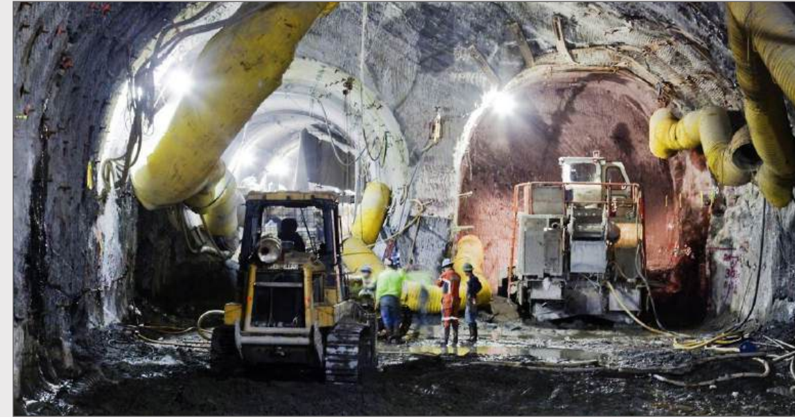
Figure 4-22 TBM Excavation Widening for Cavern Development
