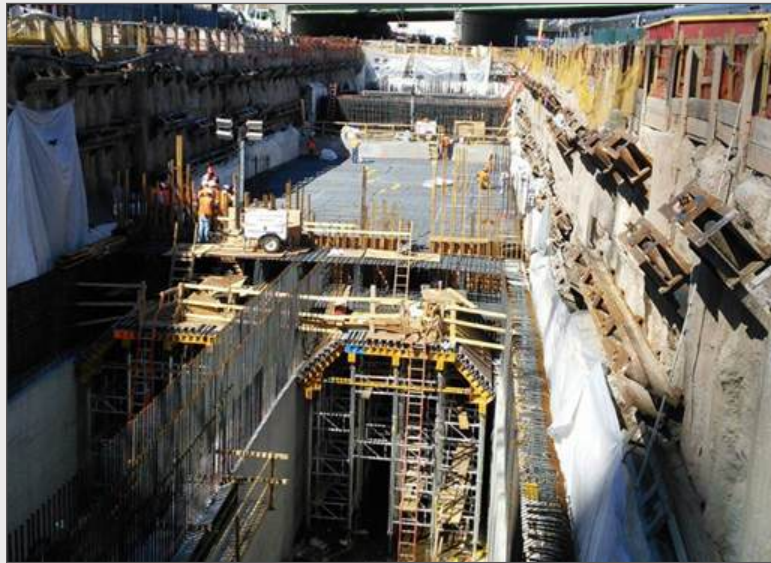
Figure 4-28 Hudson Yards Concrete Casing Project
