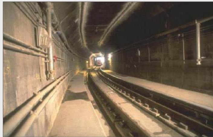
Figure 4-5 Empire Tunnel (Amtrak)
